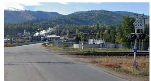
It's only safe to cross the railroad at Wisconsin, though people frequently cross at other points in the downtown area.
