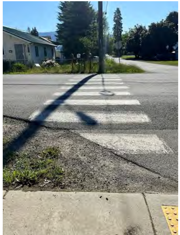
Crosswalks on 4th Street end in ditches.
